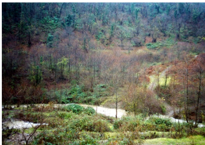
Fig. 1. Karneba River landslide, left slope (photo by S. Gorgijanidze 2001) [2].
